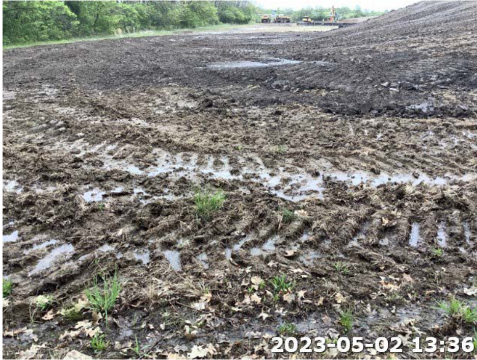
Photograph Location 7. Representative view of recently graded area within the Project area. Photograph taken facing east.
