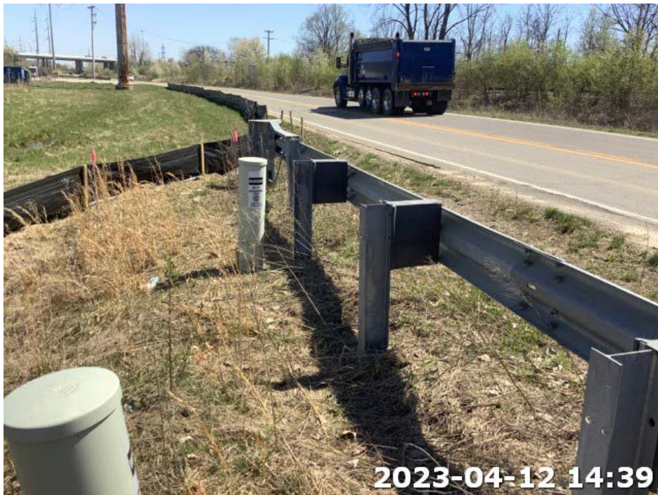
Photograph Location 6. View of upland (maintained lawn and existing paved road) at wetland determination sample point location SP06. Photograph taken facing east.
