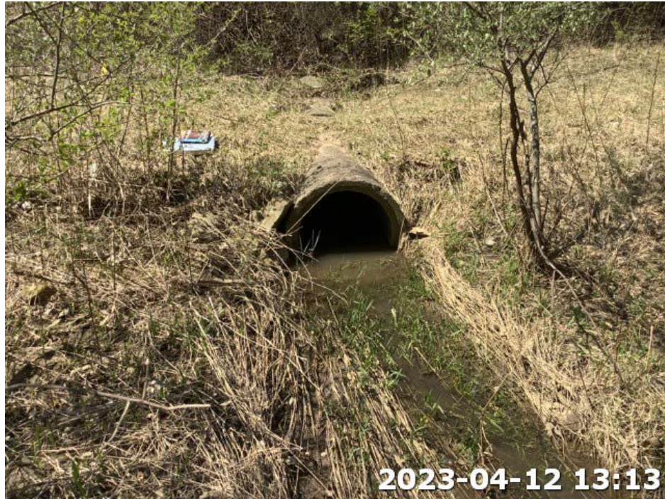
Photograph Location 14. View of existing culvert and downstream portion of Stream 1. Photograph taken facing upstream/west.
