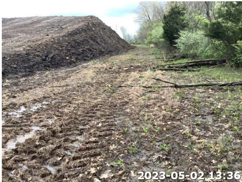
Photograph Location 27. View of upland (recently graded area) at wetland determination sample point location SP12. Photograph taken facing south.
